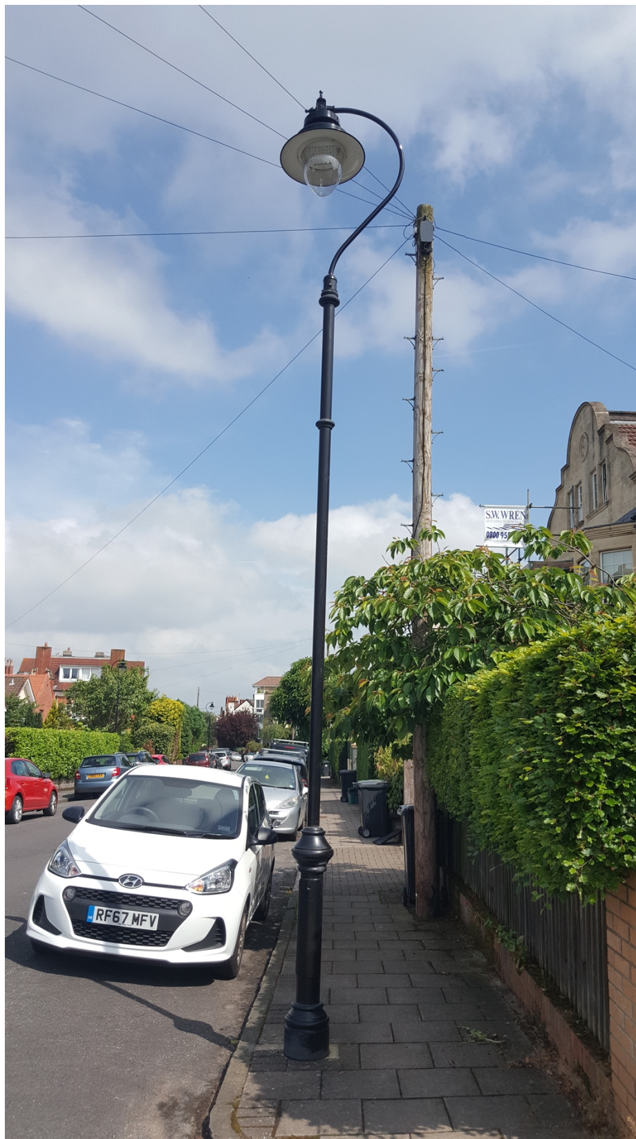
Photo H – Modern Galvanised Steel Lamp Column with Embellishment Kit
