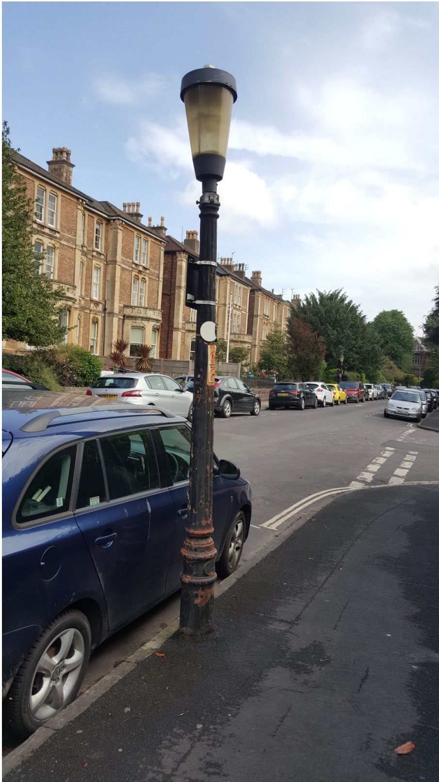
Photo C – Cast Iron Column - no door
