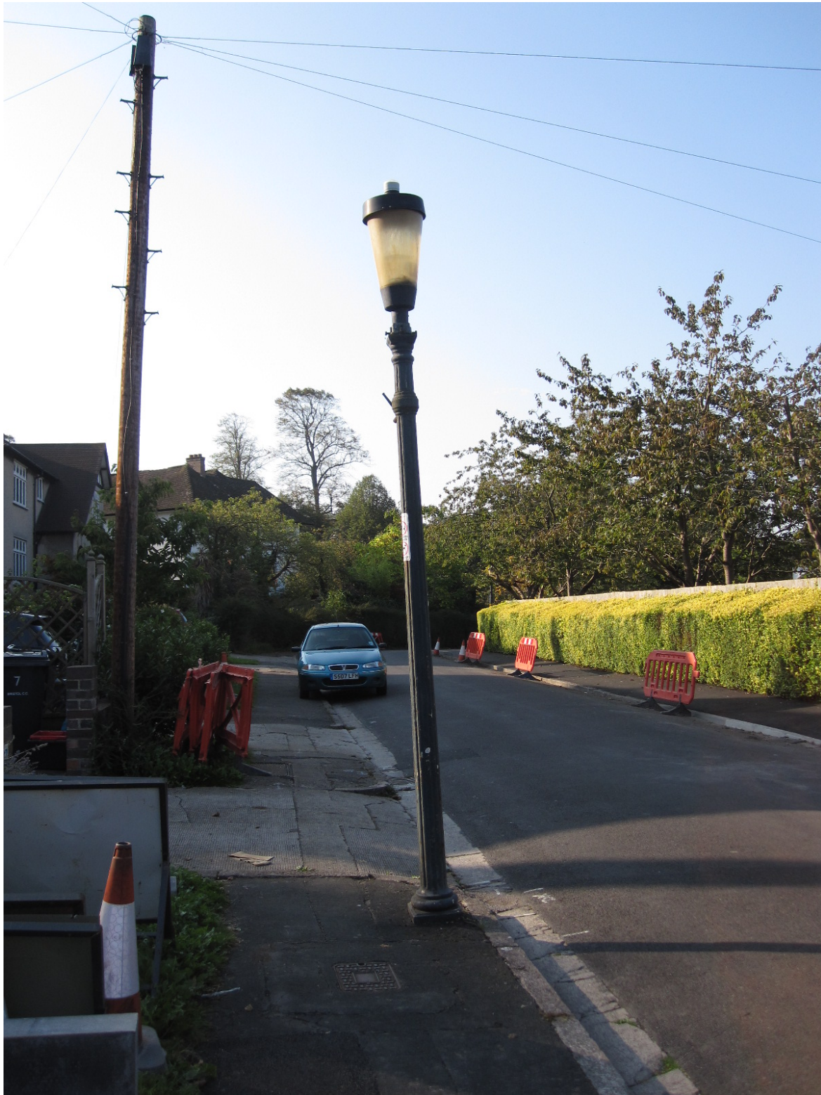
Photo B – Cast Iron Column - no door
