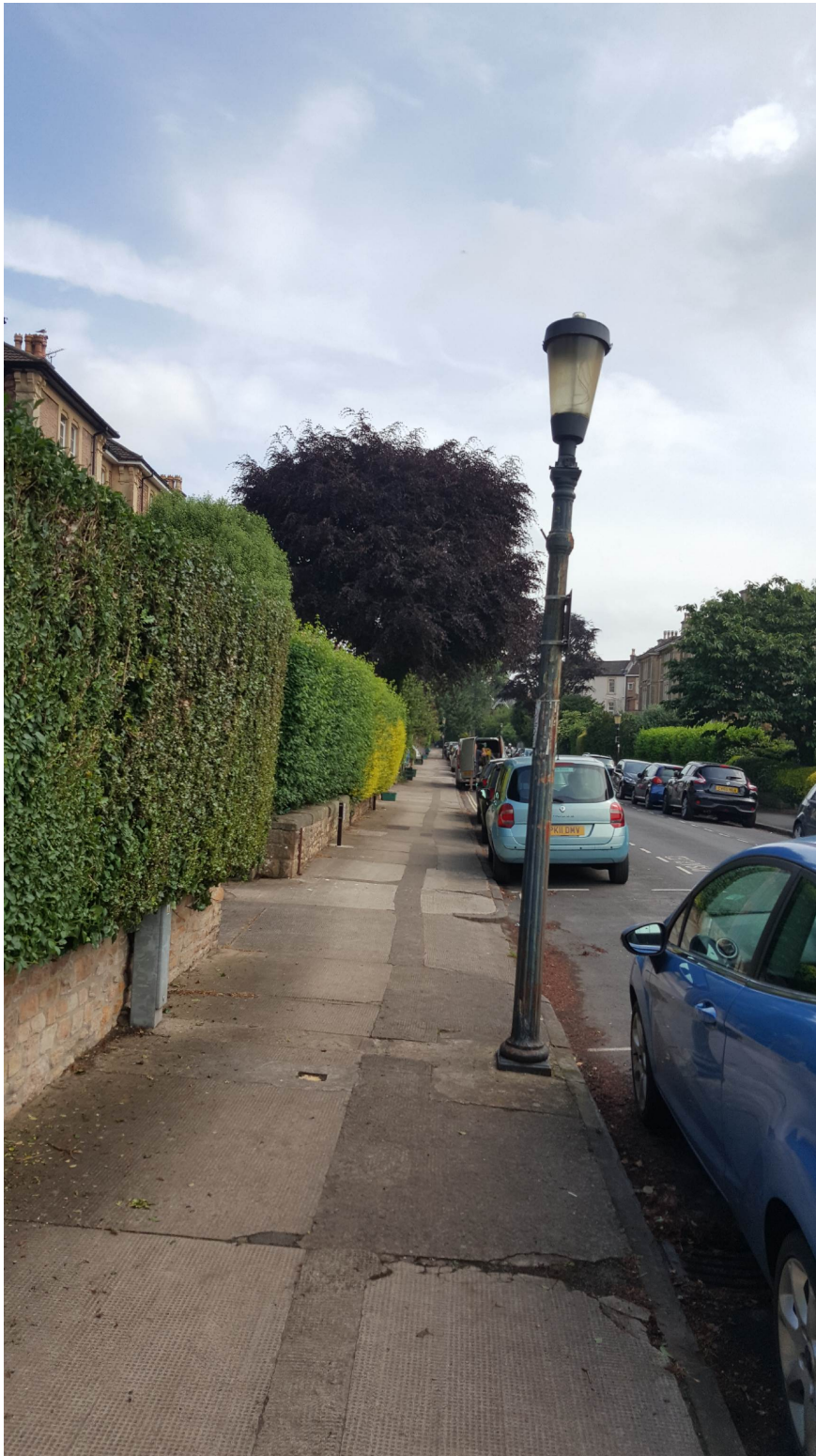
Photo E – Cast Iron Column with mains at head and mini feeder pillar
