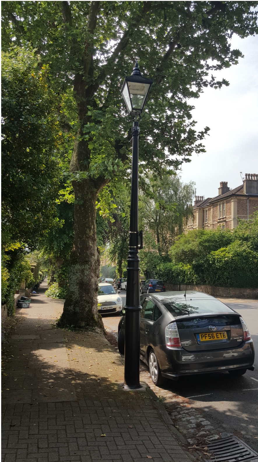
Photo D – Extended Cast Iron Column with new door access
