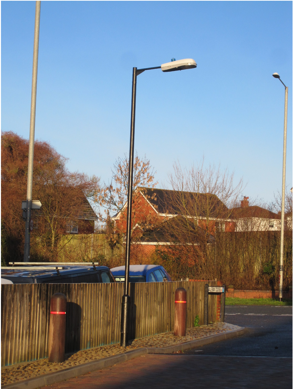
Photo G – Modern Galvanised Steel Lamp Column
